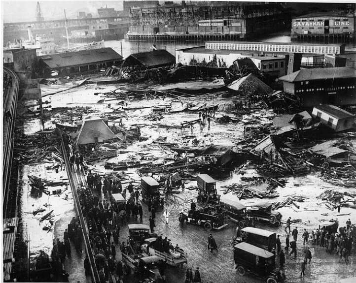
Figure 1. Aftermath of molasses tank failure
